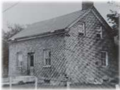
Curate's House 1967 before stucco
